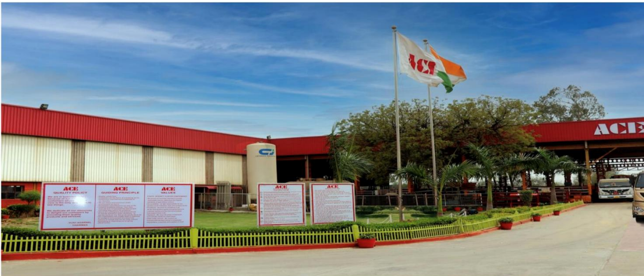
Fabrication Unit and Weld Shop
